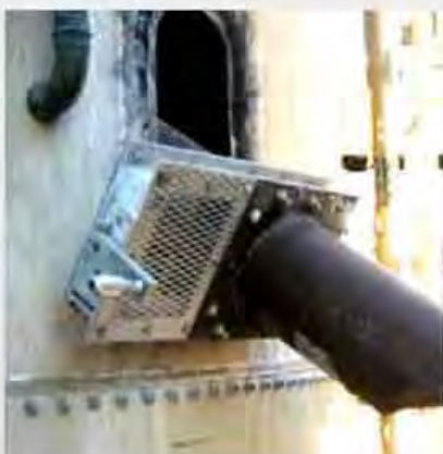
8" (203mm) Maintenance Gate utilized as overflow shutoff on silo
