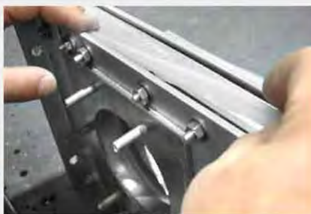
Shim removal for seal adjustment while valve is in-line
