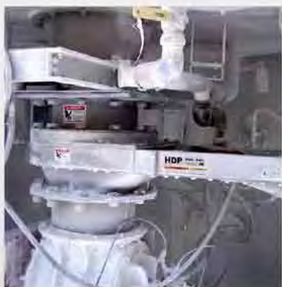
16" (406mm) HDP above airlock handling calcium oxide
