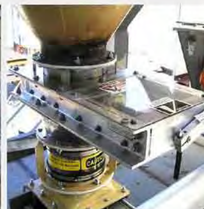
10" (254mm) Maintenance Gate handling PVC resin
